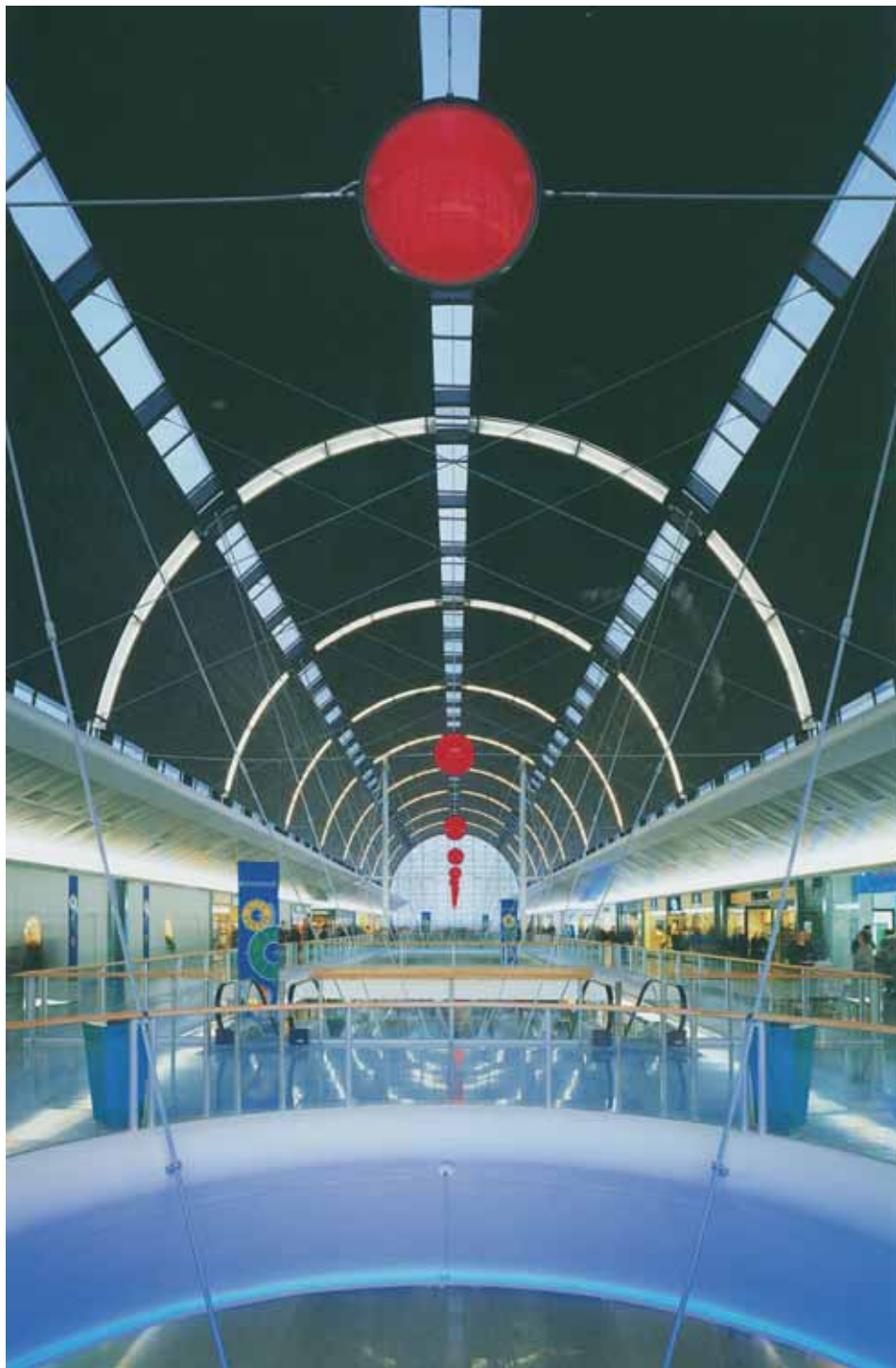
• Channel Tunnel-French Terminal, particolare interno, Calais, Francia 1986-95.
