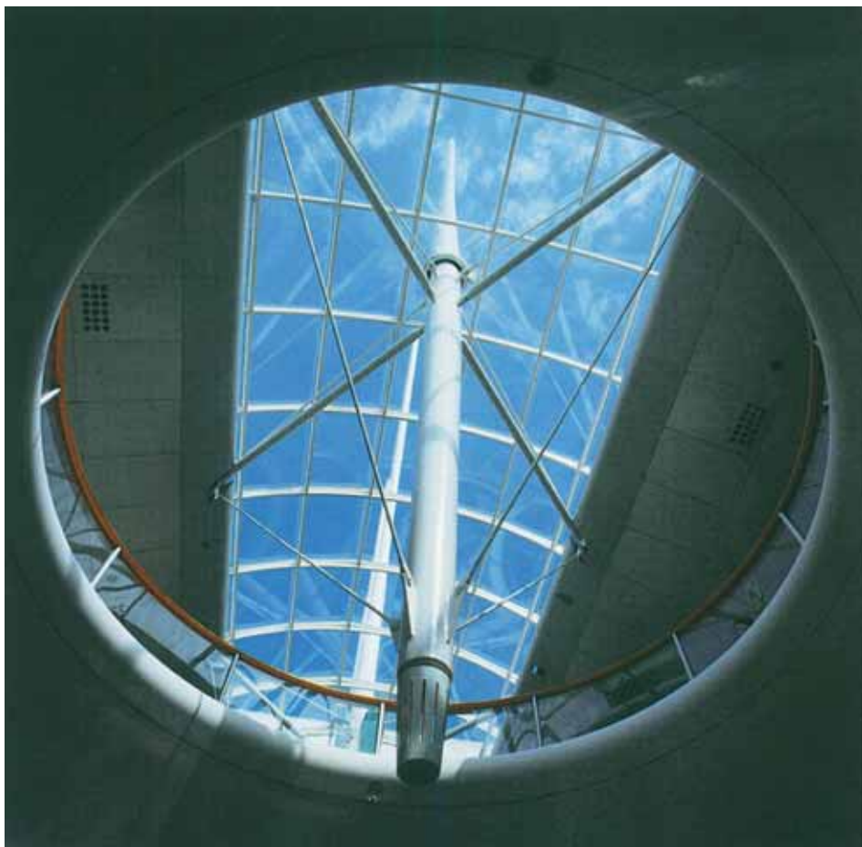
• Channel Tunnel - French Terminal, particolare, Calais, Francia 1986-93.
